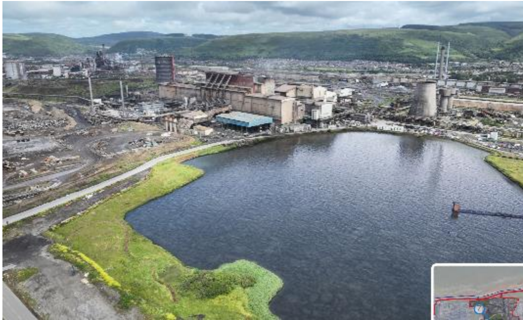
Figure 12: Lagoon and BOS Plant Existing
