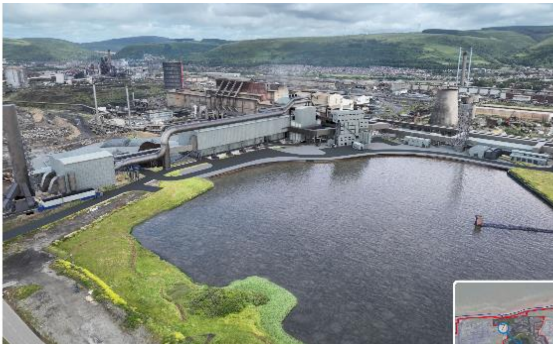
Figure 13: With EAF, Consteel Conveyor, and Fume extraction System.
