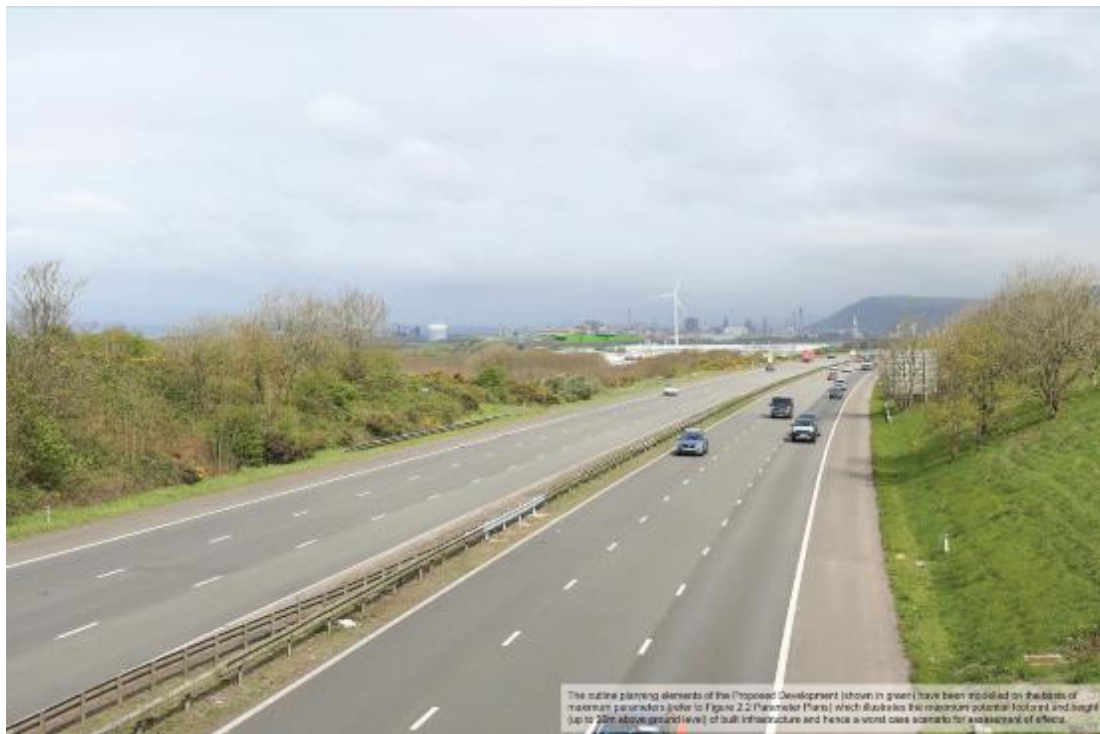
Figure 15: (ES Figure 12c) M4 Overbridge view
