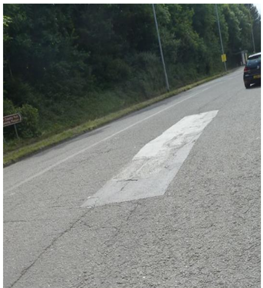
IMAGE 8 – Overbanding Example, Margam Interchange Roundabout.
