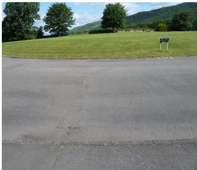
IMAGE 7 – Deterioration in Wheel Track.
