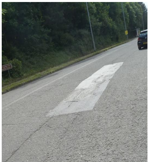
IMAGE 8 – Overbanding Example, Margam Interchange Roundabout.
