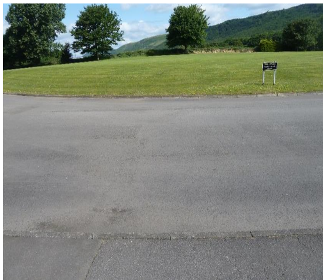
IMAGE 7 – Deterioration in Wheel Track.
