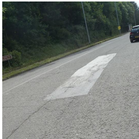
IMAGE 6 – Overbanding Example, Margam Interchange Roundabout.
