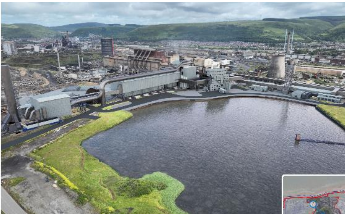
Figure 13: With EAF, Consteel Conveyor, and Fume extraction System.
